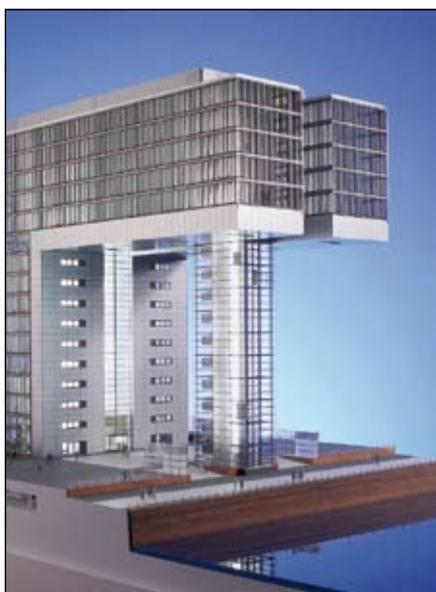
■ Kranhaus (Crane Building), Cologne scaled at 1:100; Architect: Bothe, Richter, Teherani, Hamburg; Materials: Plexiglas, polystyrene, wood (ground)
